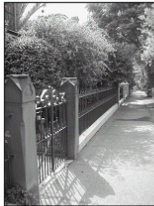
RECOMMENDED: New fencing shall complement the established rhythm of bays and openings, created by existing original fence features found in the street. Blank walls disrupt this rhythm and should be avoided.
