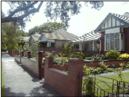
The arrangement of front fences, gardens, front and side boundary walls, pavement and trees are important stylistic features in conservation areas and must be considered when proposing new development.
